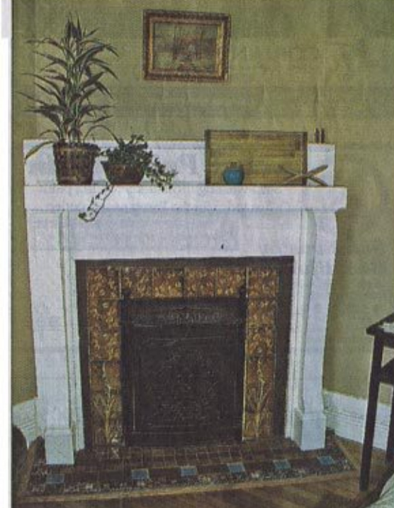
This fireplace is in the downstairs guest room. It has antique encaustic tiles on the hearth and Victorian ceramic relief tiles on the surround. The mantel is original to the house.
